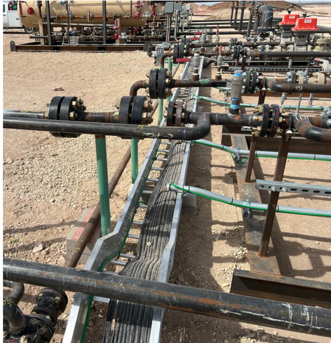
Injection Meter Skid Connection to ANSI 600 Flanged Injection Line
