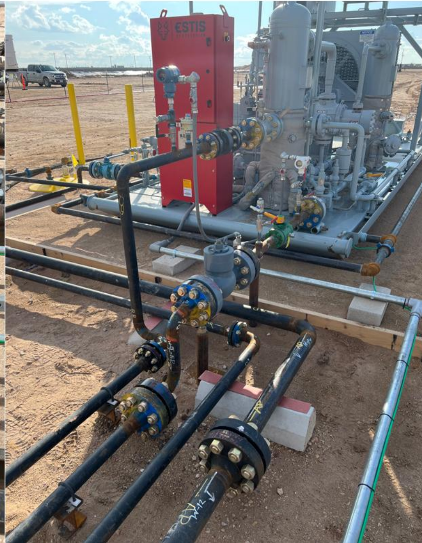
Injection Line Connection to Compressor
