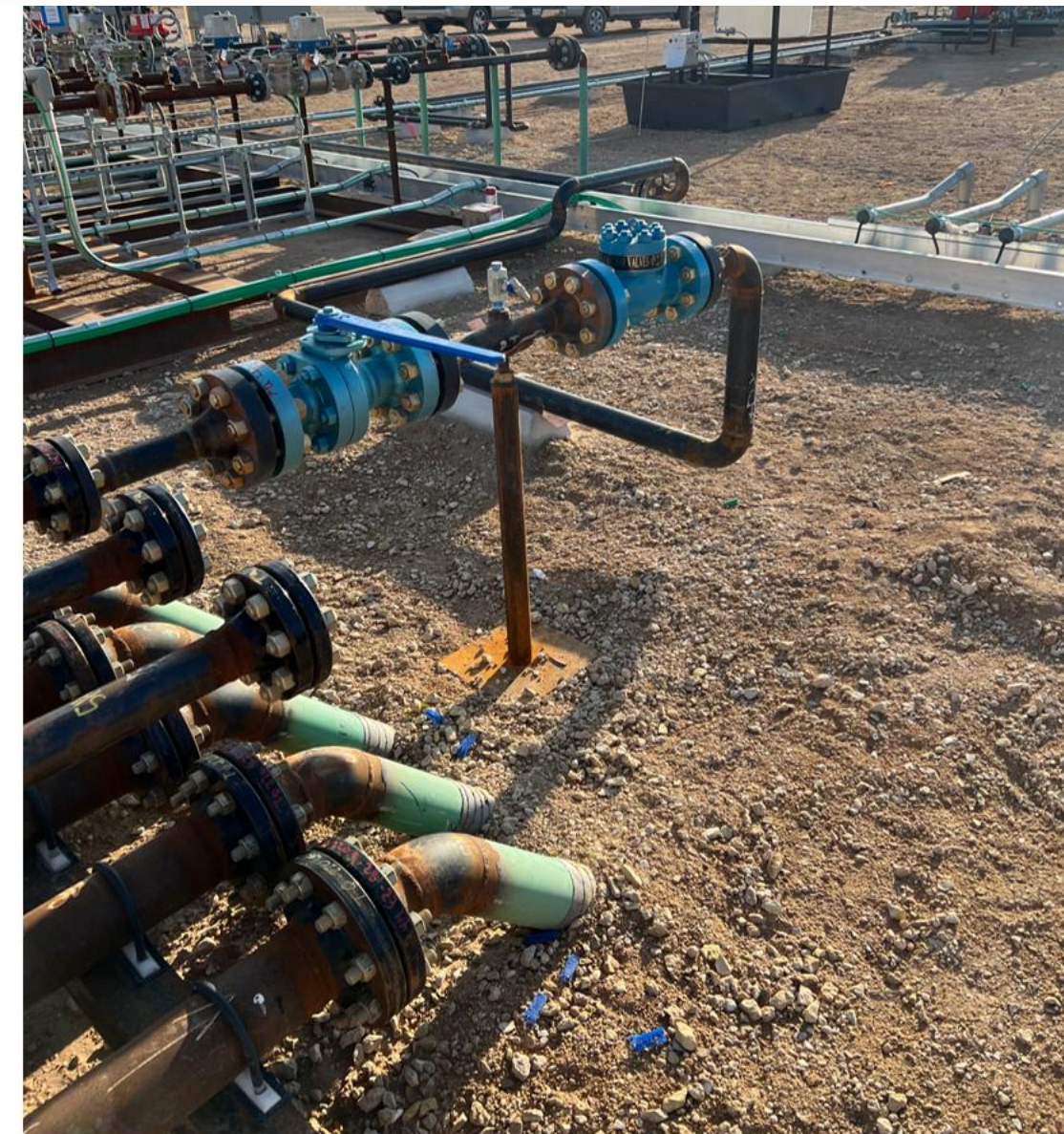
Liquid Dump Line to Flowline
