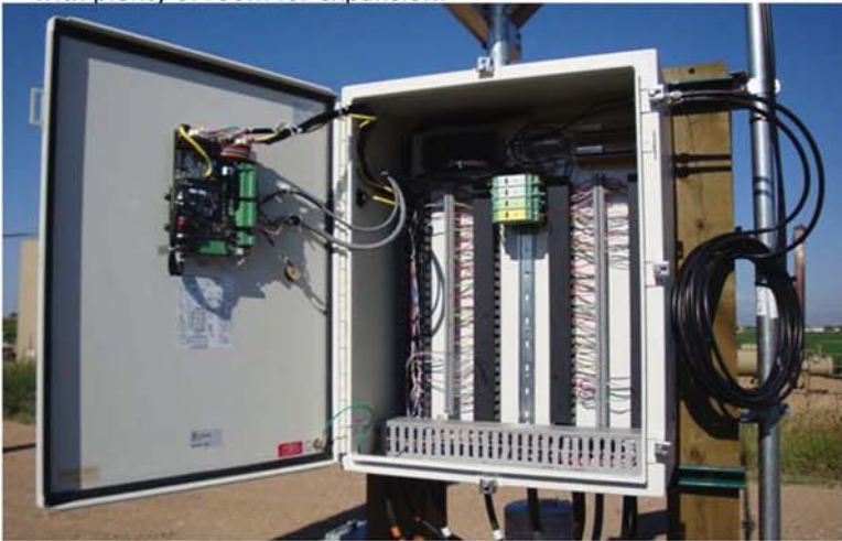
Wellhead Automation Water Pit Level Sensor Flow Line Pressure Sensor High Level Shut Down Switch ECD Temperature Sensor
